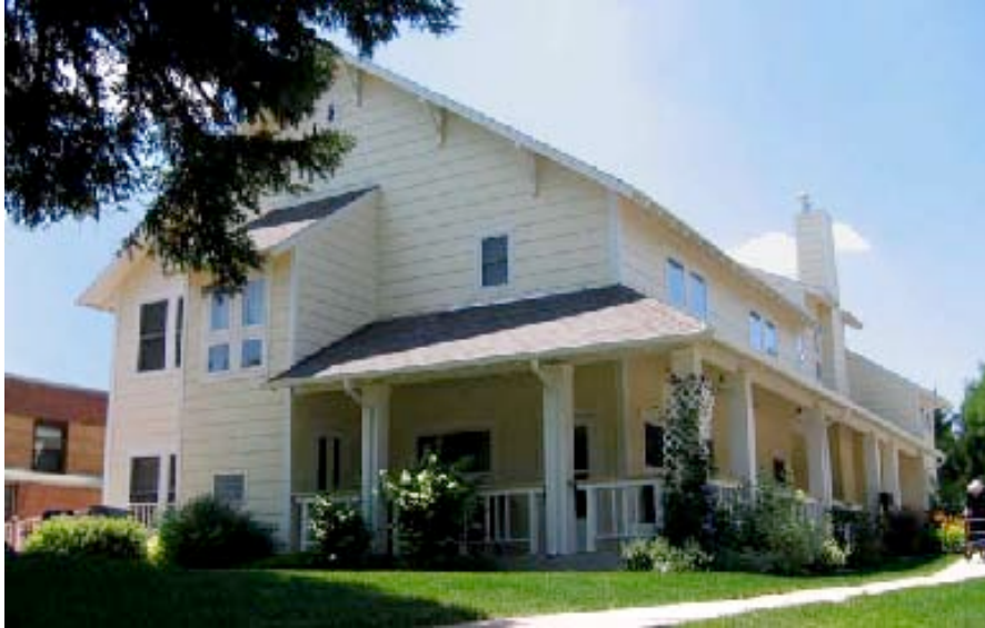
Home-like outdoor porch area for seating and reflection. Source: Campnerl & Brummett, 2010. Used with permission.
