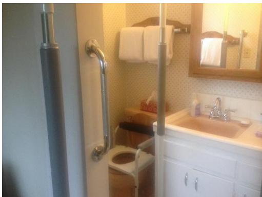
Transfer poles and grab bars support independence and safety. Source: Author.
